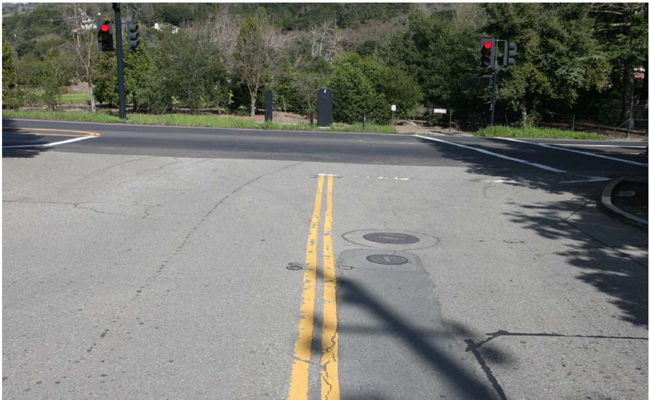
Clarmount Avenue PCI 80
