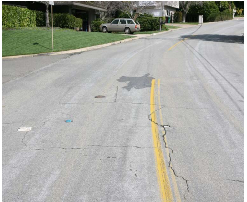
Ardith Drive at Darnby PCI 47
