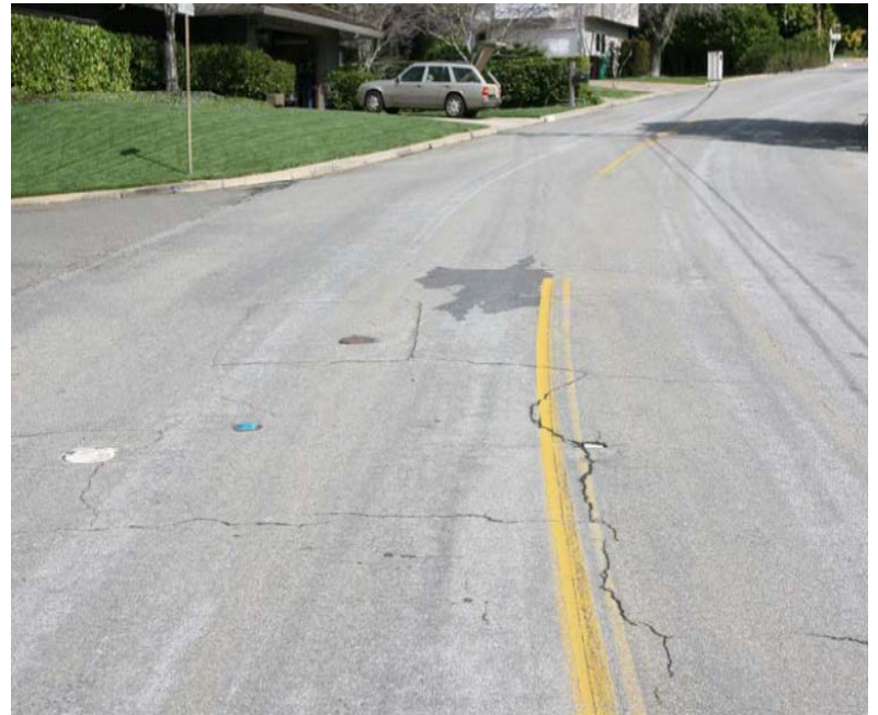
Ardith Drive at Darnby PCI 47
