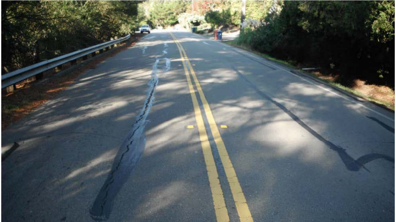
Rheem Blvd PCI 70
